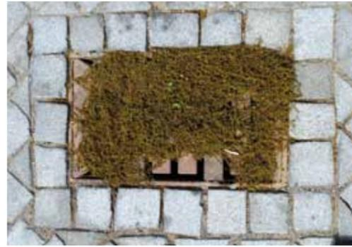
Figure 16: Limited function of the street inlet caused by rain-wash of plant material, here on the Trammplatz in front of the New Town Hall.
